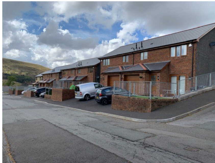
Photograph 2 – Showing site as viewed from the south western corner of the site.
