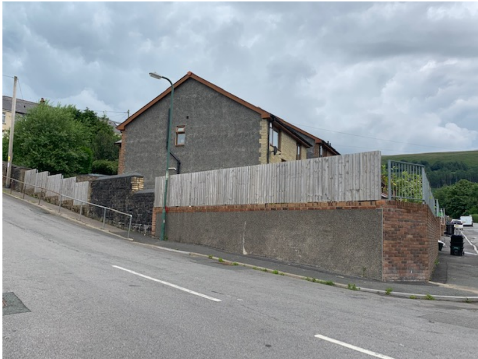
Photograph 9; Photograph of western boundary finishes where only a small section of the former school wall has been retained and the railings have been removed and the boundary has been demarcated by a rendered wall and close boarded fencing.
